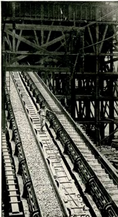
TWO OF THE IMMENSE PAN CONVEYORS AT THE PORTO BELLO PLANT
